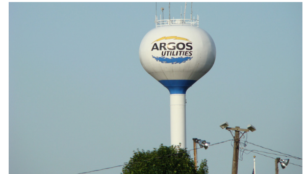
Town of Argos Water Tank
